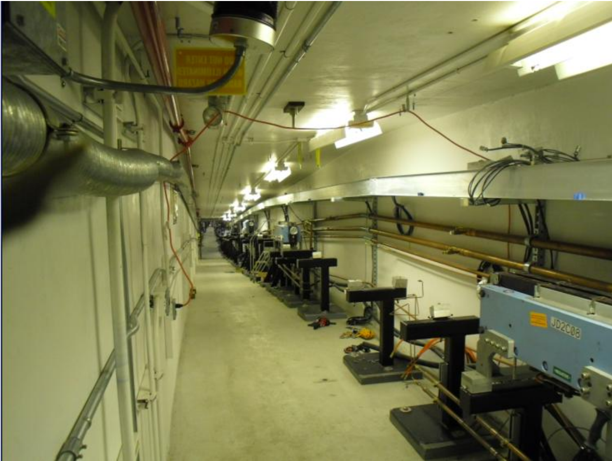
2C quad girders removed
